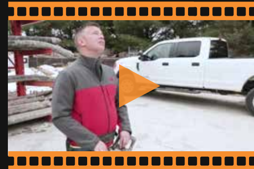
Concrete Pumping (Filmed).
